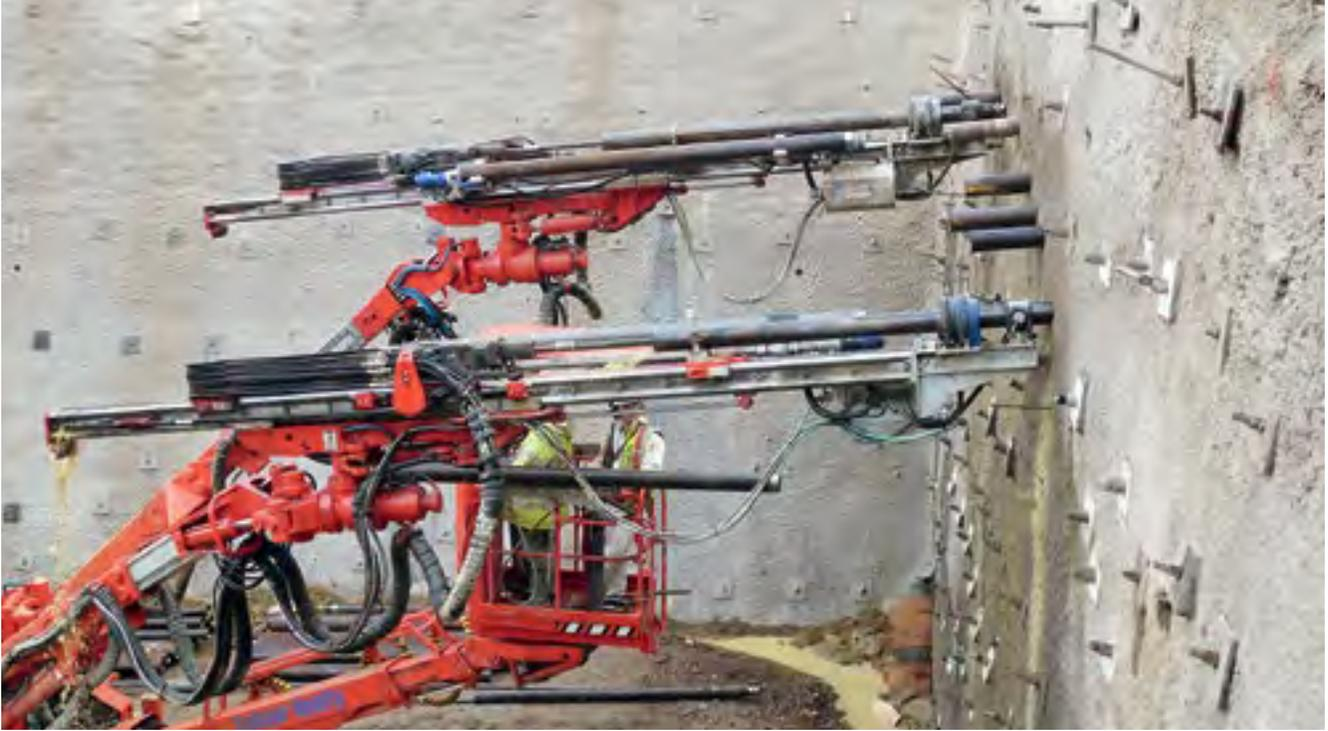
1. For drilling, the starter unit with drill bit is assembled onto the drill boom together with the first extension tube, the adapter, and the drill rod.
