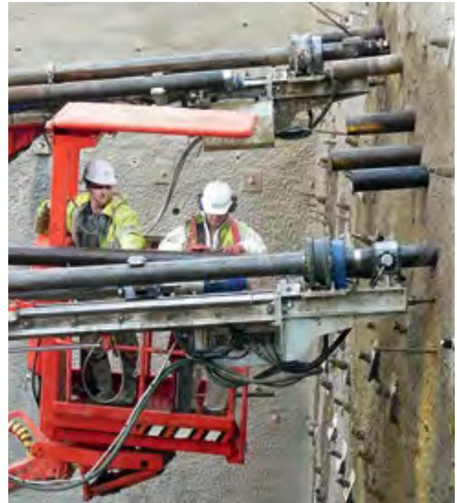
4. The last step is to be repeated until the designed length of the AT – Pipe Umbrella has been installed. Followed by removal of adapter and drill steel.
