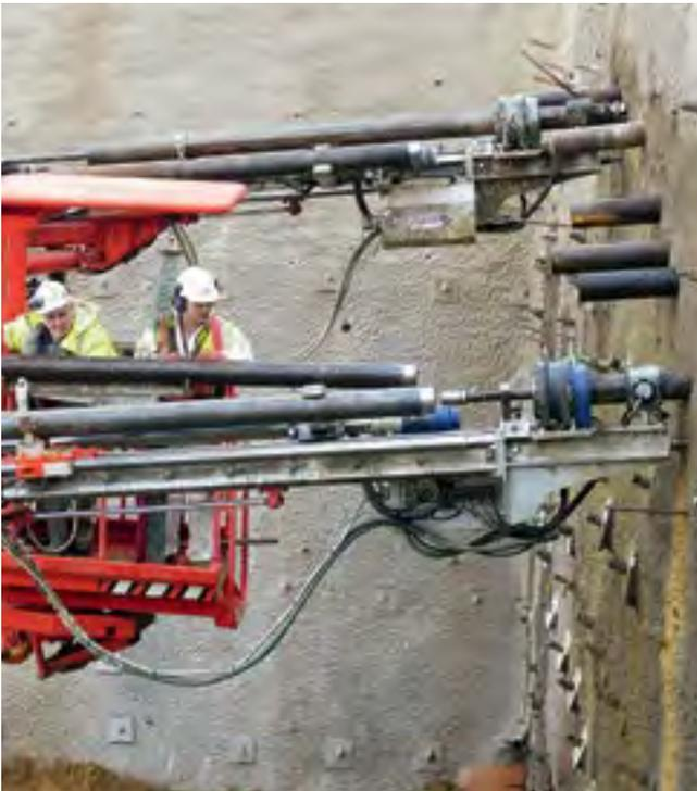
3. The next drill rod with extension tube is connected to the previously installed pipe and the drilling process is continued. Reloading AT – Automation Unit (extension tube and drill rod).
